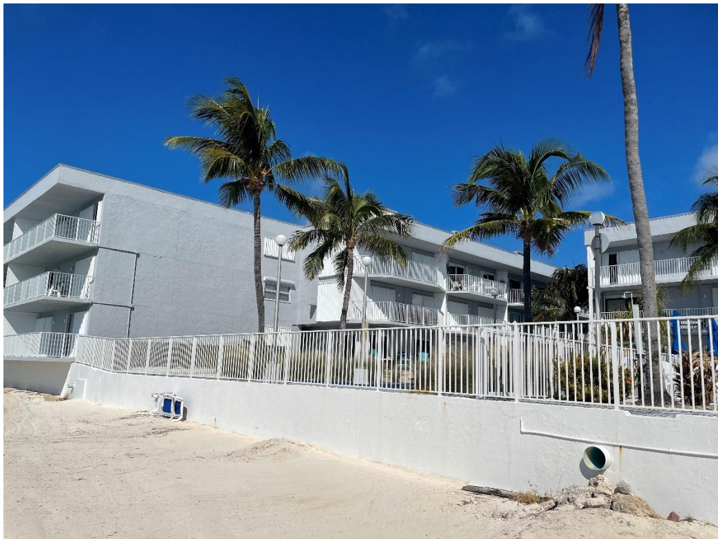
Photo #6 - Overview of Buildings #3 (left) and #2 (right)
