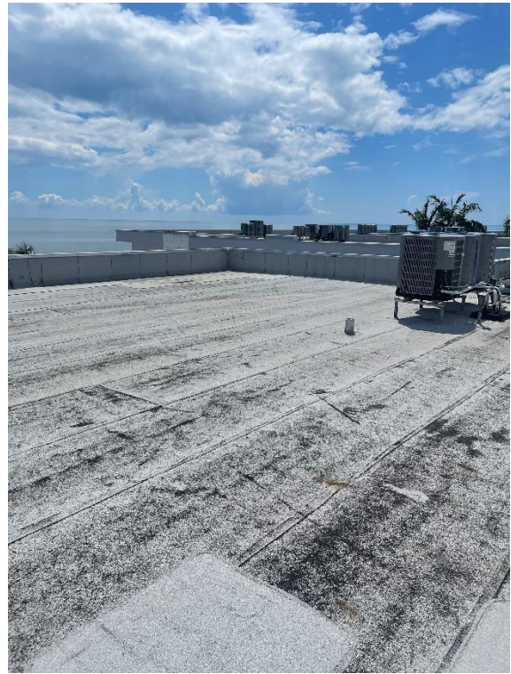
Photo #16 - Overview of Roof
