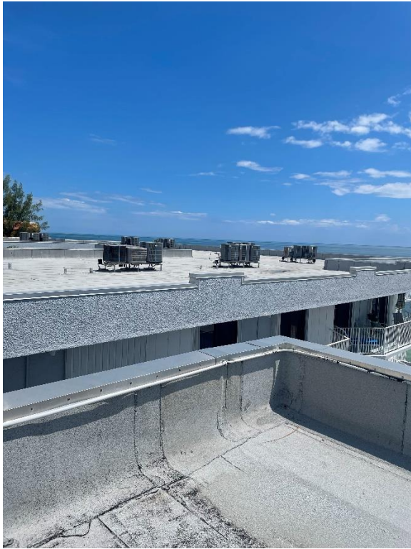
Photo #15 - Roof Corner w/ Parapet Wall Cap
