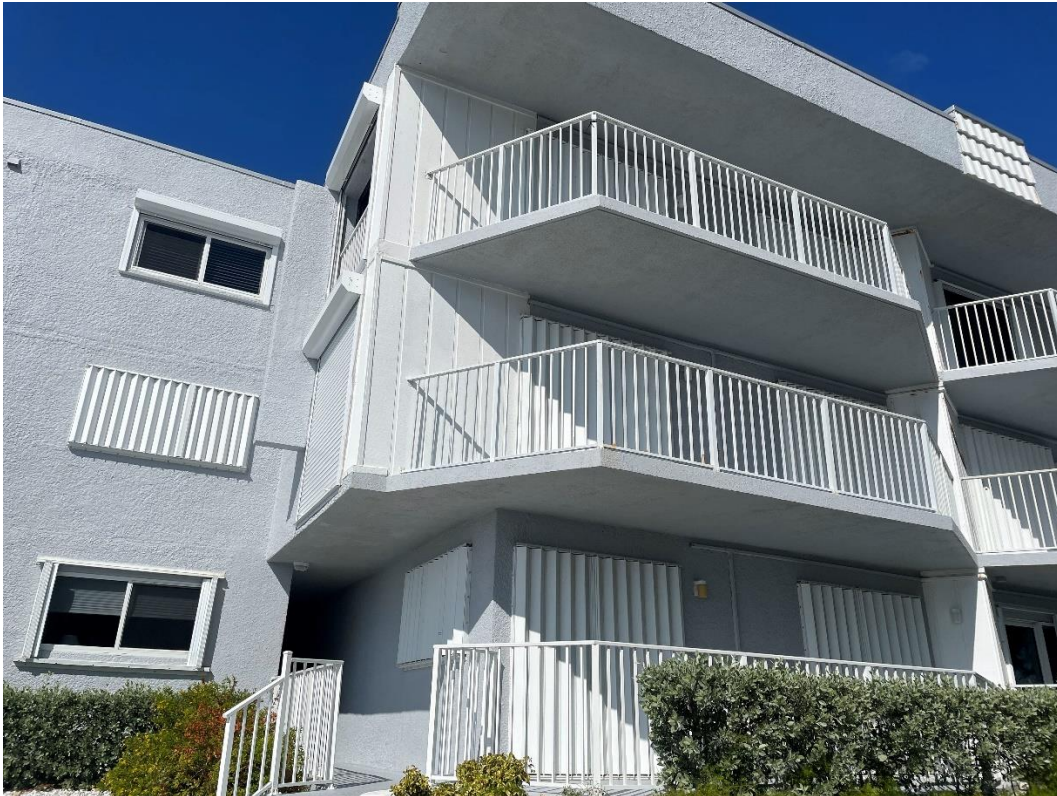
Photo #3 - Typical East and West Balconies at Buildings #1 and #3
