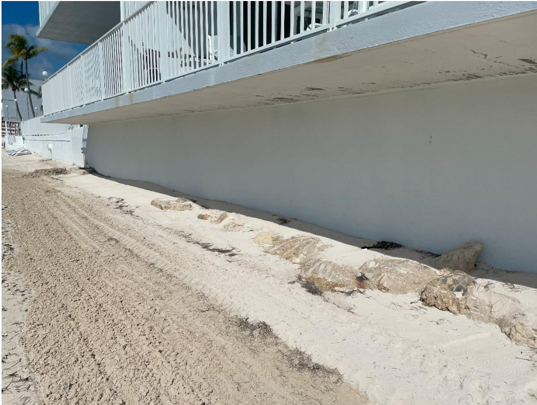
Photo #5 - Retaining Wall Below 1 st Floor – Buildings #1 and #3
