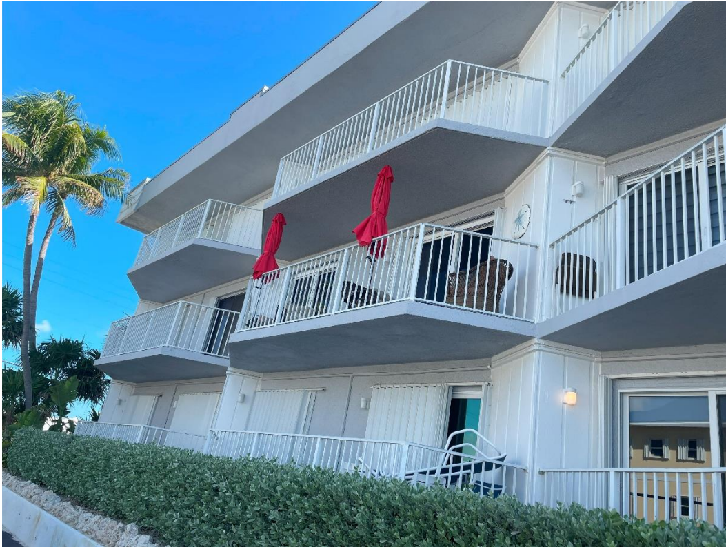
Photo #7 - Typical East and West Balconies at Buildings #1 and #3
